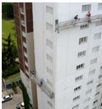
Photo 4-3 外壁の断熱改修工事 Repair Work of Façade Heat Insulation
