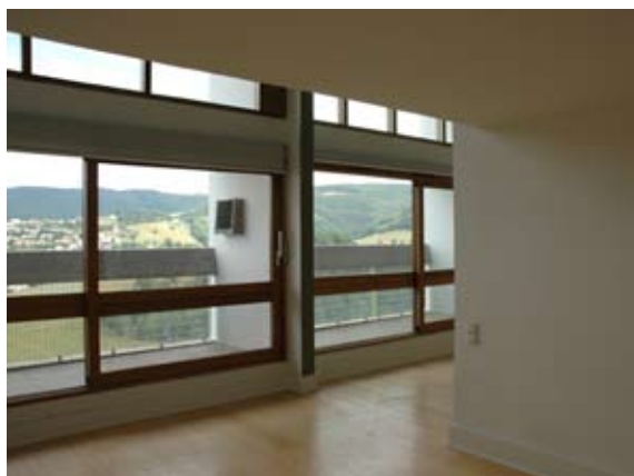
Photo 6-6 断熱遮音ガラスへの改修 Replacement of Window Glass with Heat Insulating Soundproof Glass
